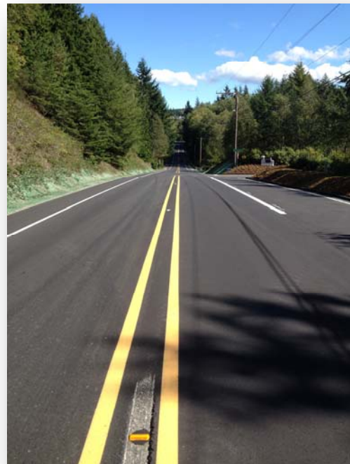
The newly rehabilitated Road provides a safe and smooth ride for residents and visitors.
