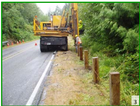
1. The intersection of Center Road and Egg & I Road before safety upgrades. 2. New, high visibility stop and street signs installed at the same intersection. 3. Driving posts for 425-feet of guardrail installation on Paradise Bay Road Milepost (MP) 2.2. 4. Newly installed guardrail along 250-feet Paradise Bay Road MP 1.9.
