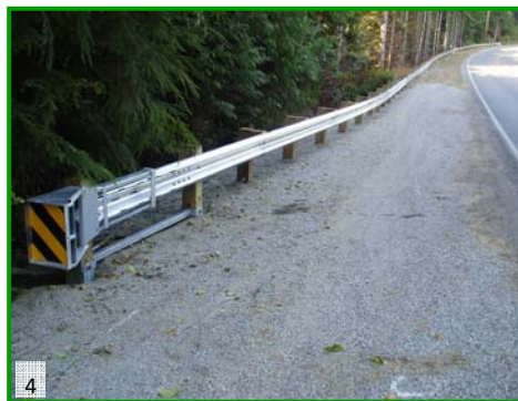
1. The intersection of Center Road and Egg & I Road before safety upgrades. 2. New, high visibility stop and street signs installed at the same intersection. 3. Driving posts for 425-feet of guardrail installation on Paradise Bay Road Milepost (MP) 2.2. 4. Newly installed guardrail along 250-feet Paradise Bay Road MP 1.9.
