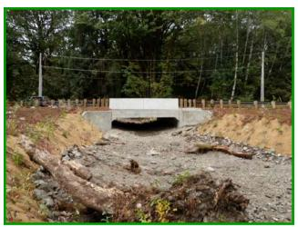
The new box culvert is 22-ft wide and 40-ft long. Other improvements to Spruce Creek included grade controls to improve streambed stability and protect the structure from scour.
