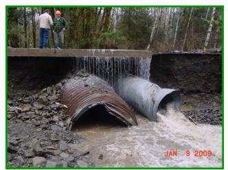
The old Spruce Creek culverts—with diameters of 72-in and 48-in — and the Upper Hoh Rd above, damaged by flooding.
