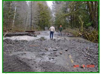
After the storm event in January, 2009, debris covered the Upper Hoh Rd and water eroded parts of the road surface.
