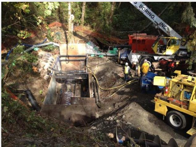
Construction crews at work during the pipe ramming phase of the project.
