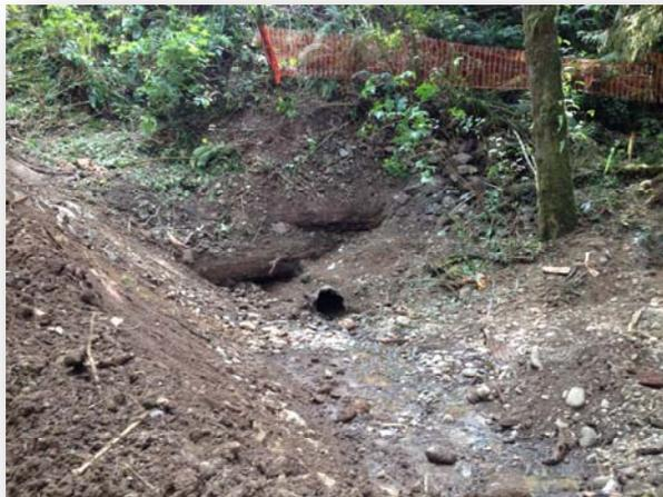
The old culvert located beneath the road embankment was severely deteriorated and in danger of collapsing. Inlet shown.
