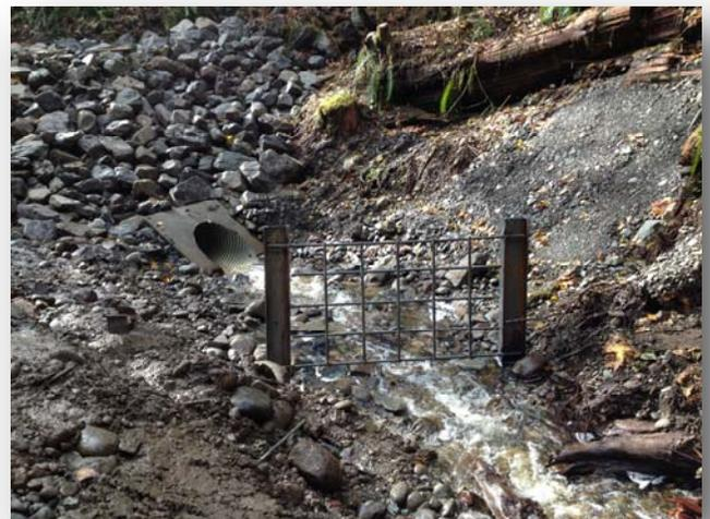
The new culvert will preserve the road integrity at this location far into the future. New inlet with concrete headwall and debris rack shown.
