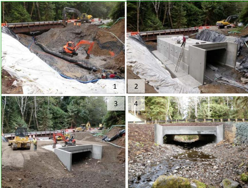
Critical steps in the culvert replacement project: 1. Excavation of the stream bed with road and stream bypasses in place and a portion of the Upper Hoh Road removed. 2. Installation of the three-sided, box culvert. 3. Restoration of the stream bed and preparation for the road re-build. 4. One mile of upstream fish habitat restored.
