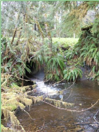
The old culvert under the Upper Hoh Road was rusted out and formed a barrier to upstream fish habitat.
