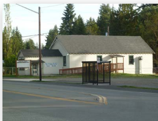
A new trail, bus pullout and transit stop improve visibility and safety for students, pedestrians and bicyclists.
