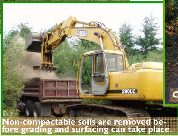
Non-compactable soils are removed before grading and surfacing can take place.
